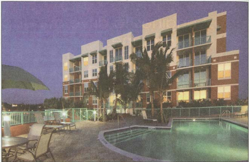
The Progresso Point rental apartments opened at 619 N. Andrews Ave. in Fort Lauderdale.
